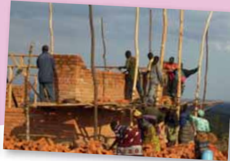
The new school under construction
