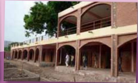
Carrefour des Jeunes, building in progress Turing Foundation Project Visit, November 2010
