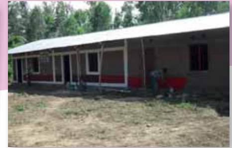
Medical school nearing completion
