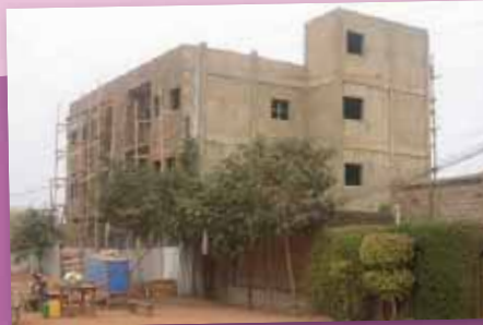
Vocational training centre CPAEC under construction
