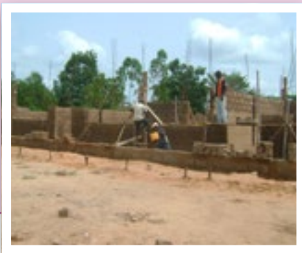
Benin Construction of a primary school, Fanta
