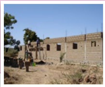
Mali Construction of a technical school in Kambila
